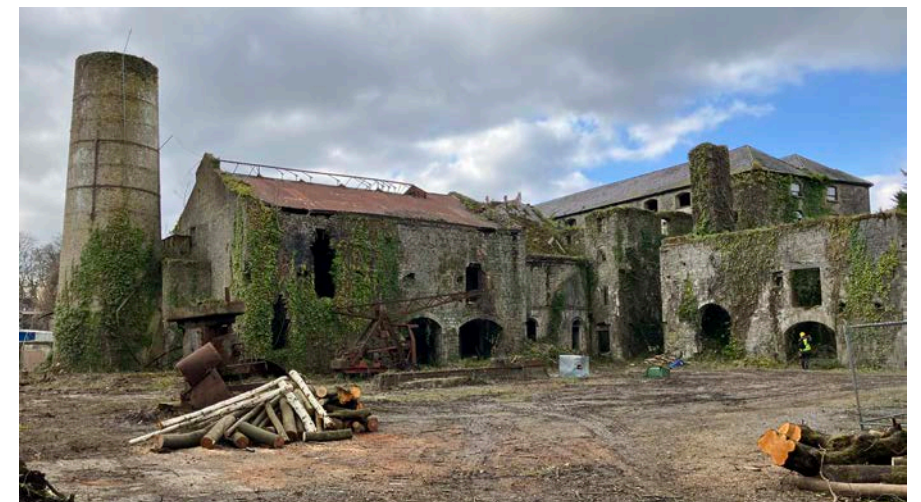
Figure 9 - Main distillery buildings from the South East.
