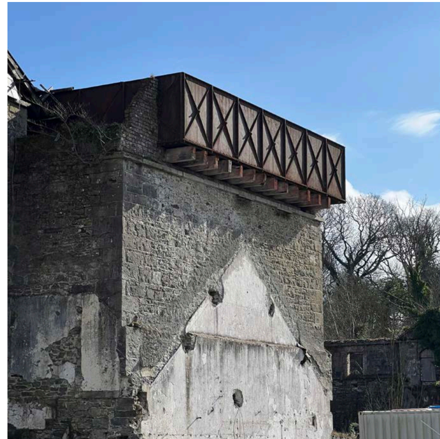
Figure 144 - Water tower from the north.
