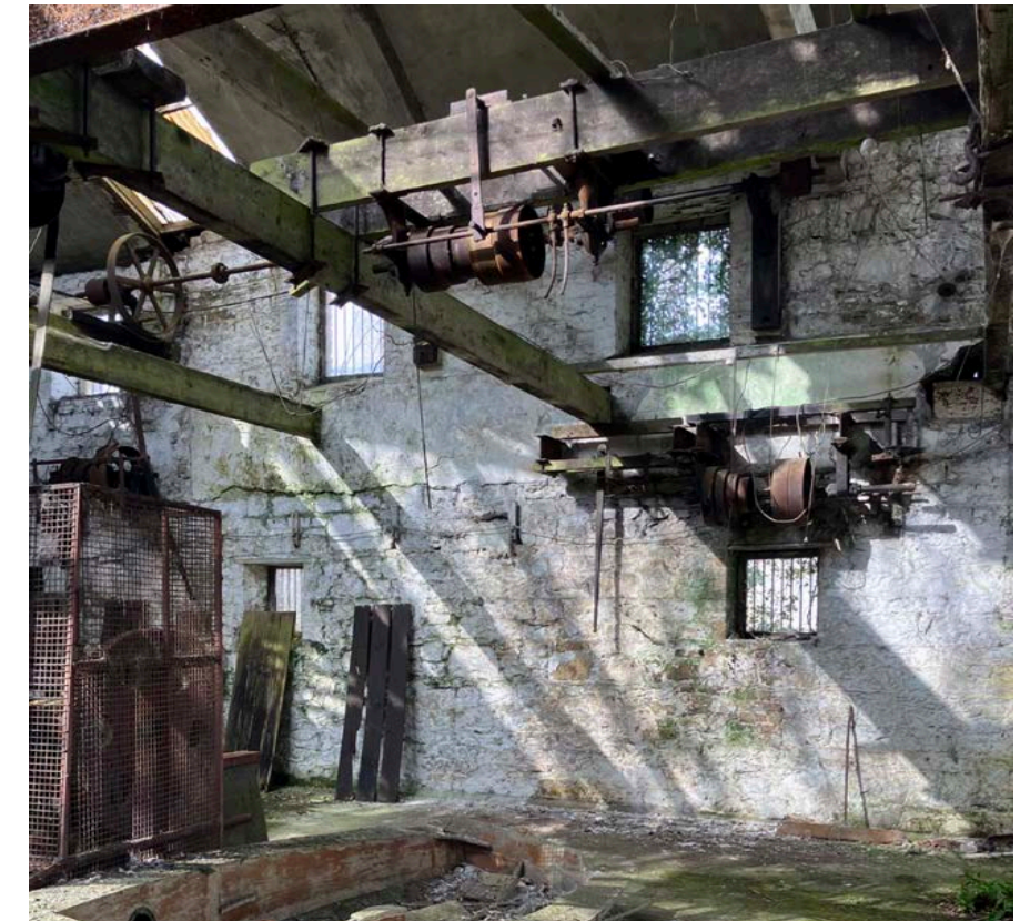
Figure 122 - Long shop - south facing opening.
