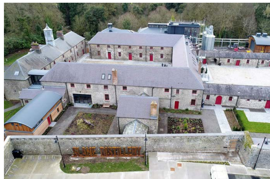
Figure 123 - Aerial view of Slane Distillery, Co. Meath.
