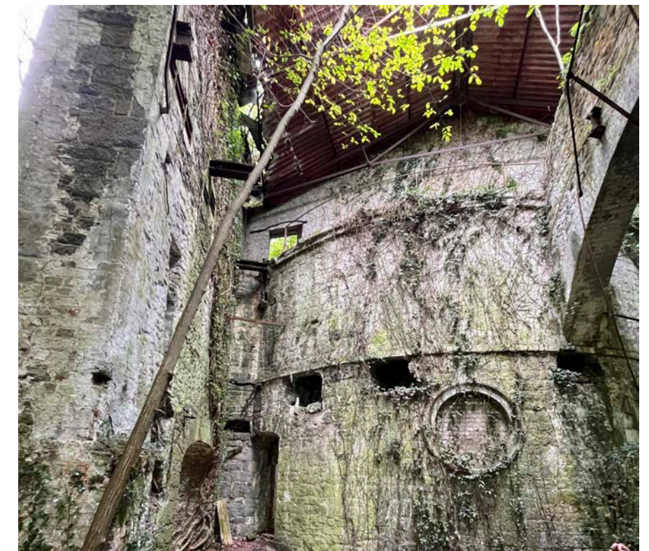
Figure 45 - Mash house looking north from inside the still house.
