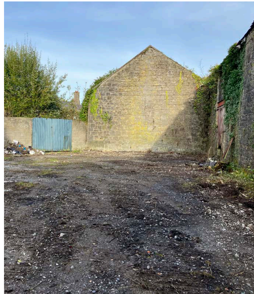
Figure 64 - View of the splayed eastern gable of the store/ workshop.
