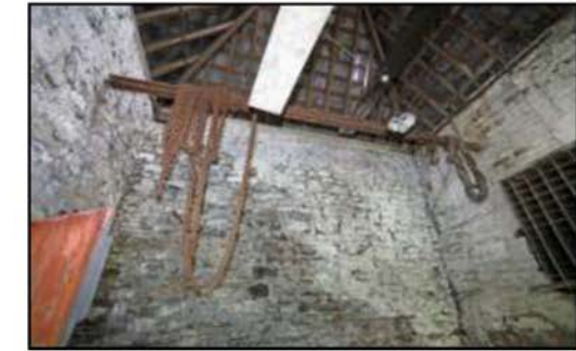
2. Hanging chains at N end of room.
