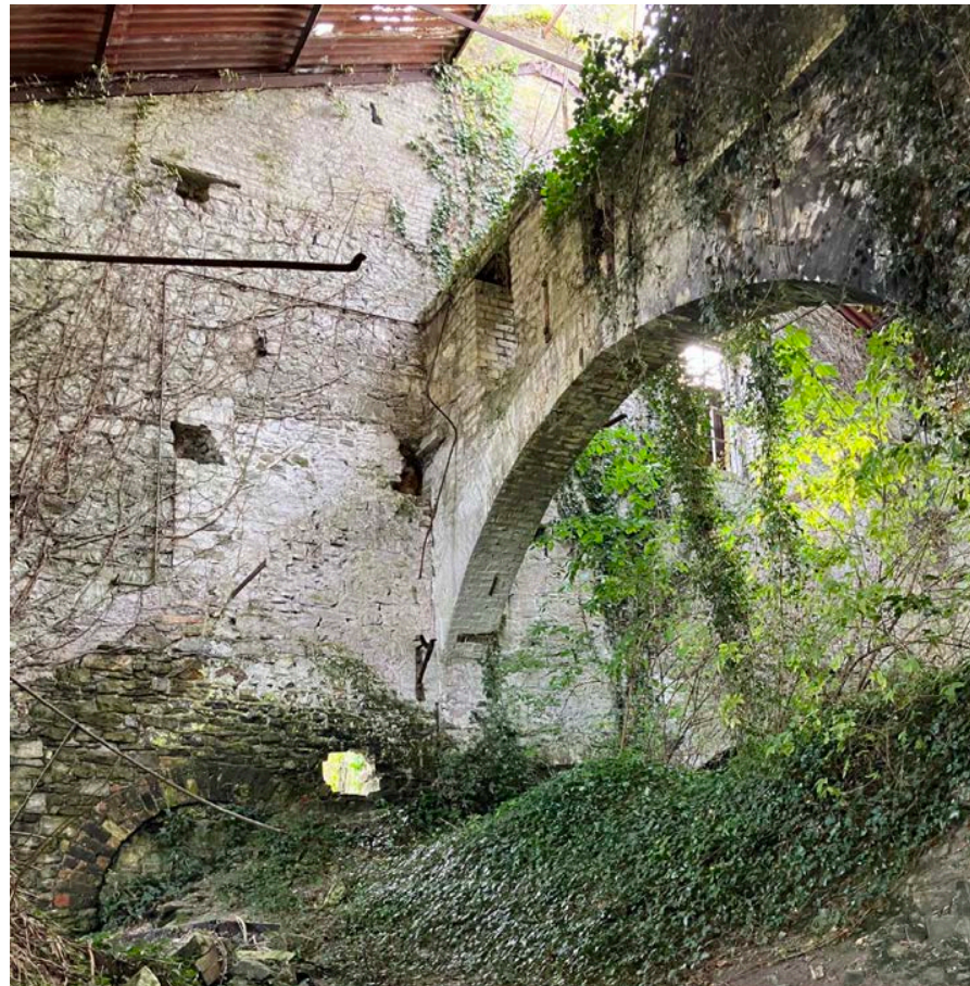
Figure 52 - Still house interior detail of flying butress.
