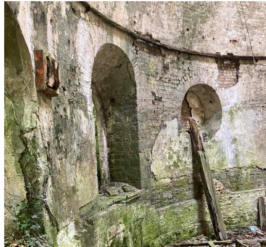
Figure 43 - Mash house general view of the interior looking south.
