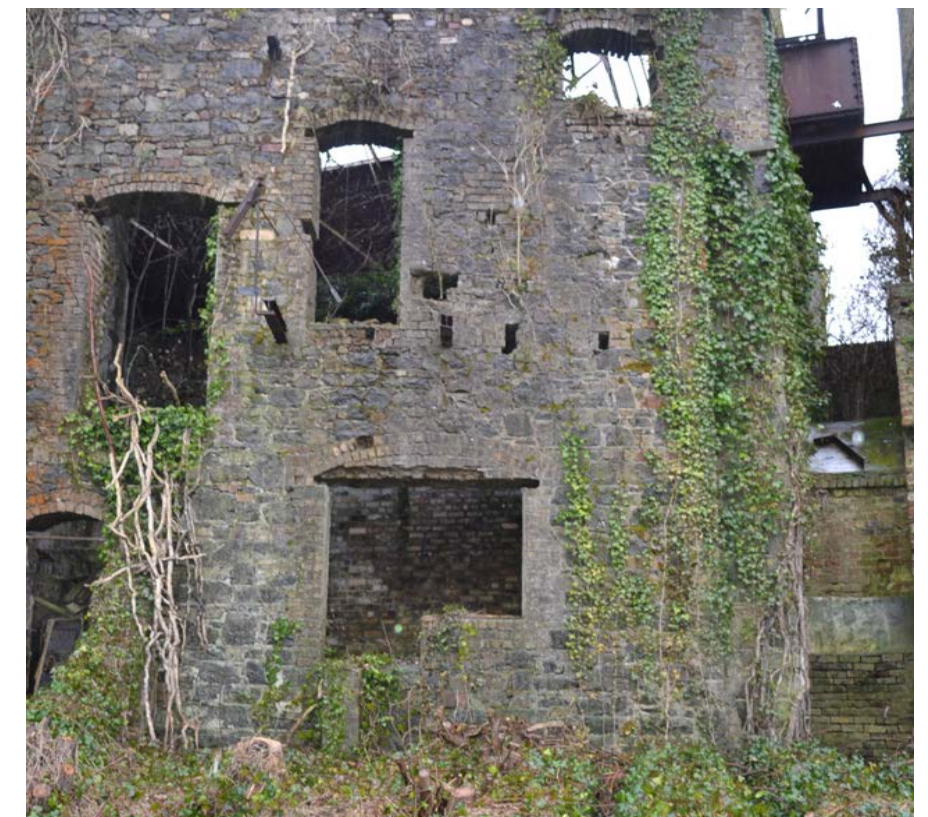
Figure 51 - Still house view from the west
