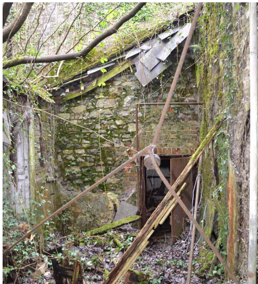
Figure 35 - Offices - roofless rear extension.
