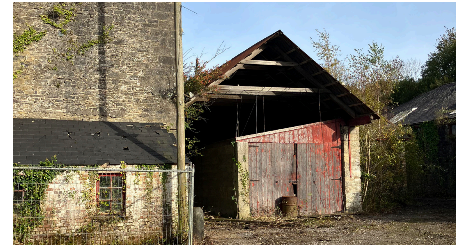
Figure 74 - Shed west end, showing pitched corrugated iron roof.
