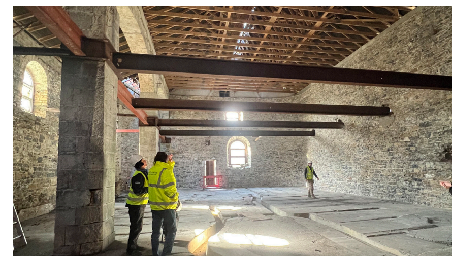
Figure 126 - Back house internal view.
