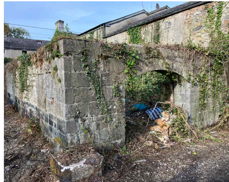
Figure 81 - Water tank masonry base beside entrance.
