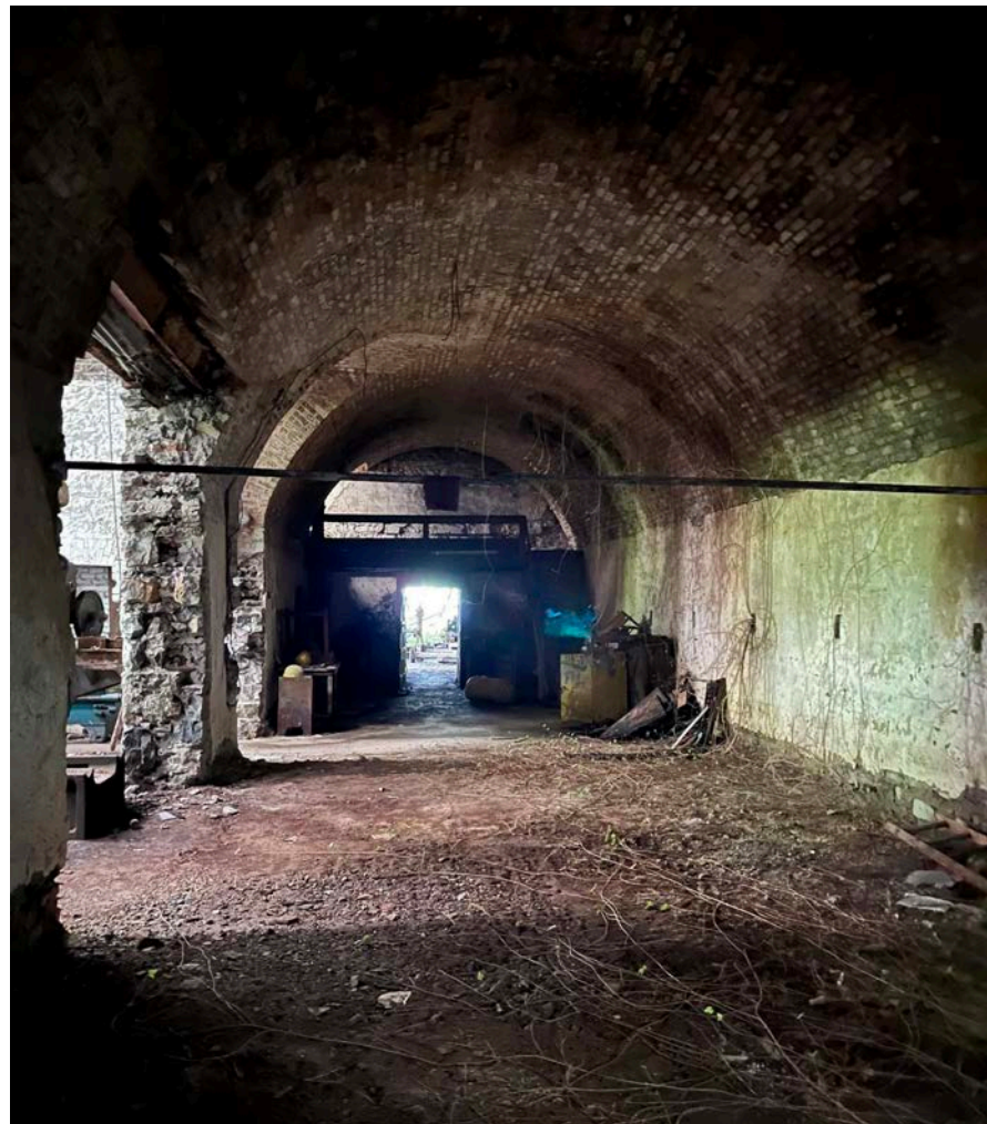
Figure 28 - Bonded warehouse looking east with removed lower floor.
