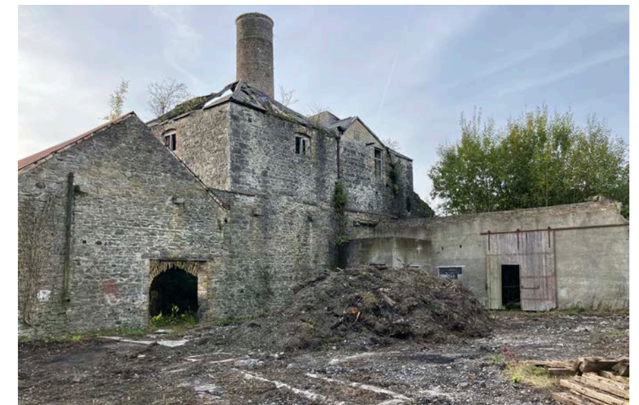
Figure 70 - Carpenters shop site behind engine house.
