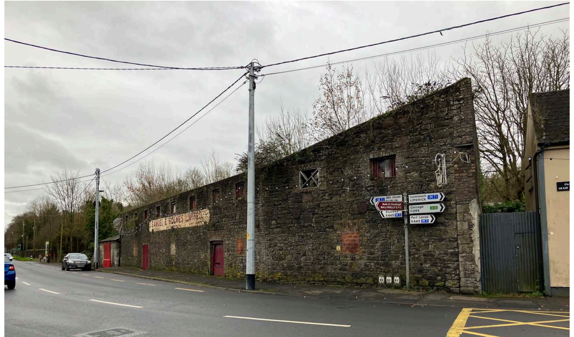
Figure 67 - Warehouse/cooperage from Dublin Road.
