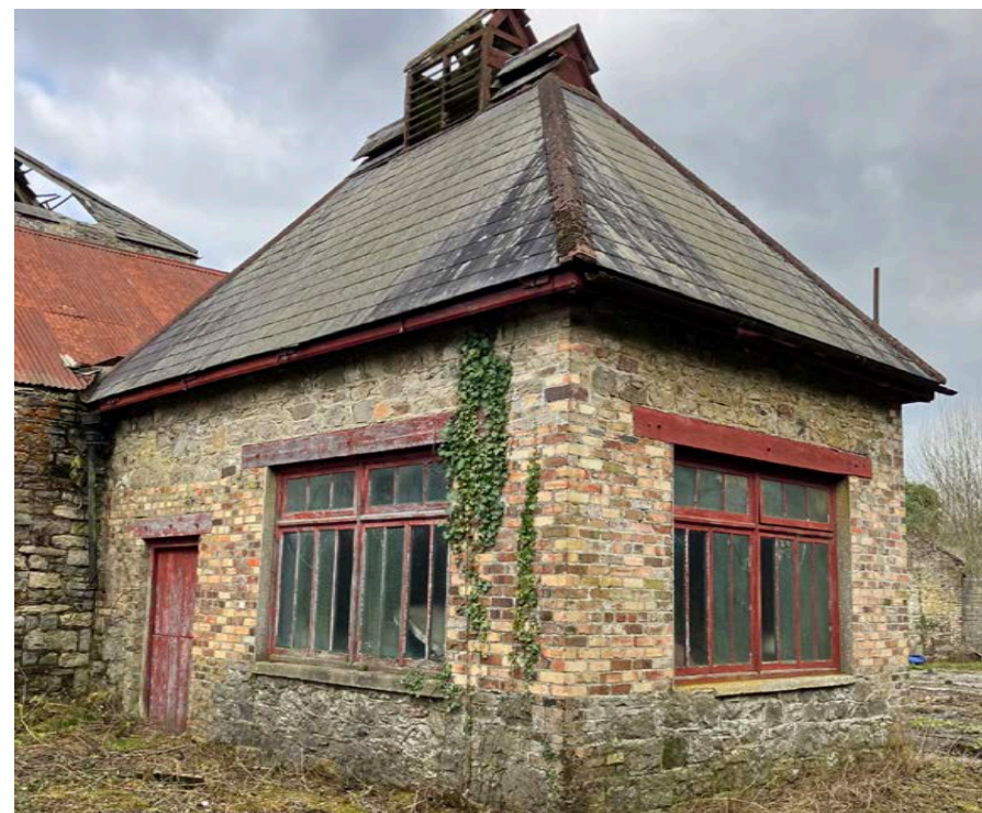
Figure 76 - Gas house general view.
