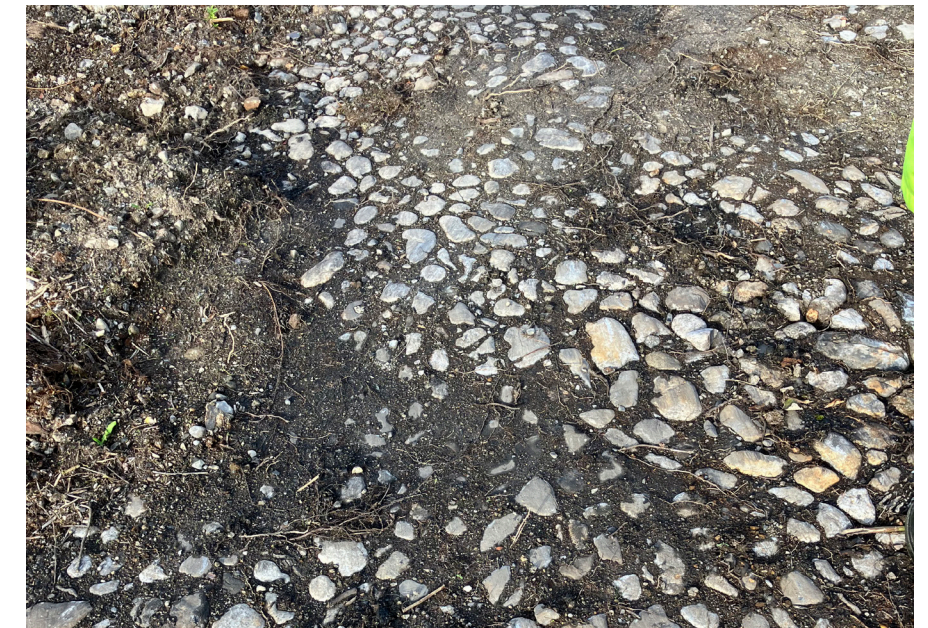
Figure 103 - Distillery yard detail of original cobbled paving.
