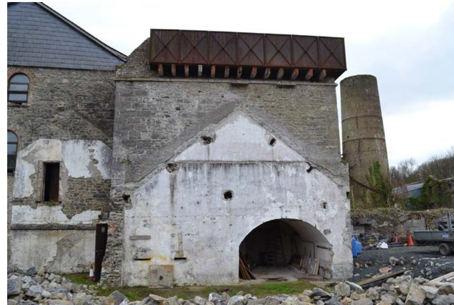
Figure 50 - Back house undercroft brick and stone vaulting.
