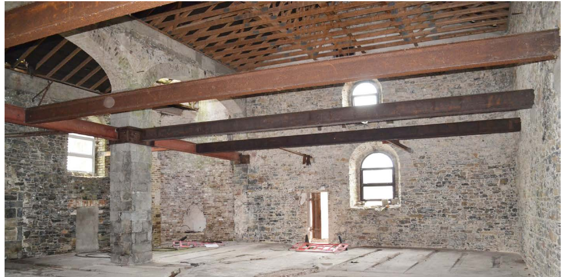
Figure 47 - Back house interior view.
