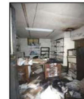
6. Interior of office, to S.
