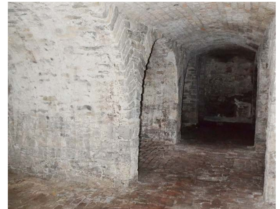
Figure 48 - Back house undercroft brick and stone vaulting.
