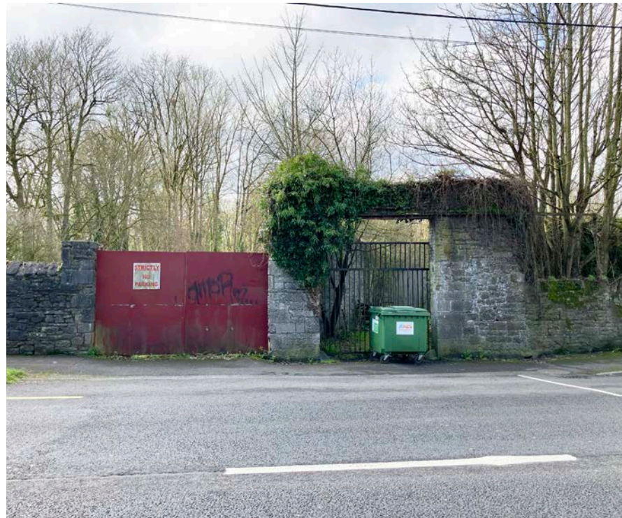
Figure 118 - Site entrance from the east off Dublin Road.
