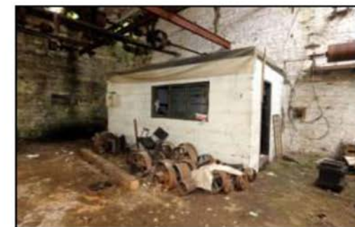
5. Office at W end of building.
