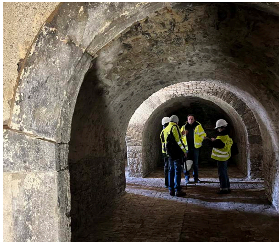
Figure 94 - Mill & grain store - infilled carriage arch.
