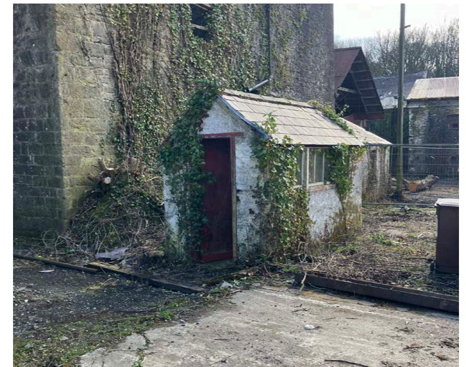
Figure 79 - Weighhouse external view.
