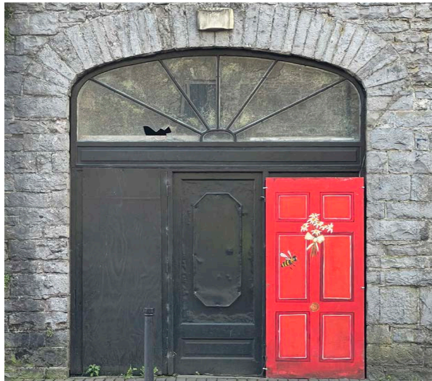
Figure 141 - Mill & grain store infilled carriage arch.
