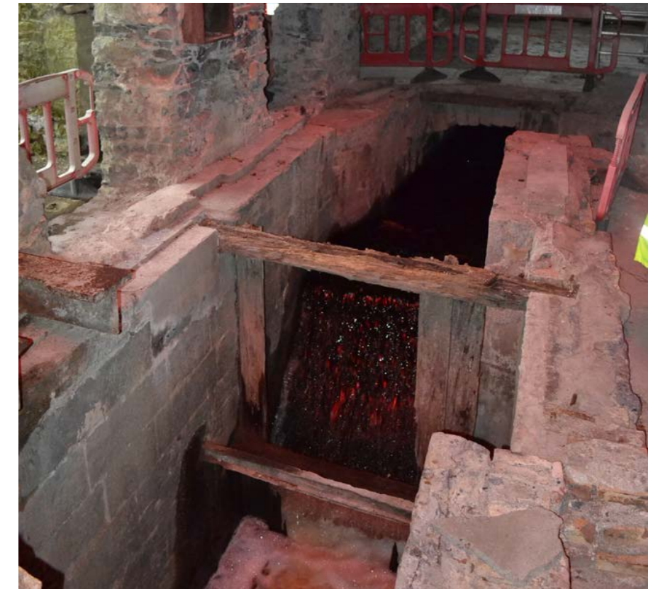
Figure 40 - Mill and grain store likely waterwheel location.
