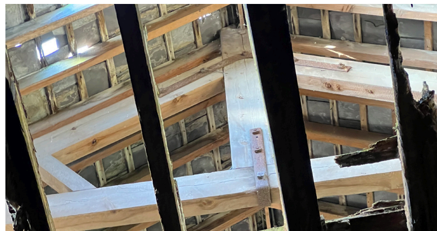
Figure 84 - Malt house king post roof trusses.
