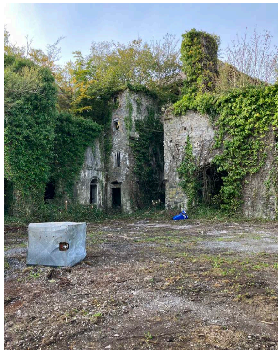
Figure 36 - Former engine house invaded by trees and shrubs.
