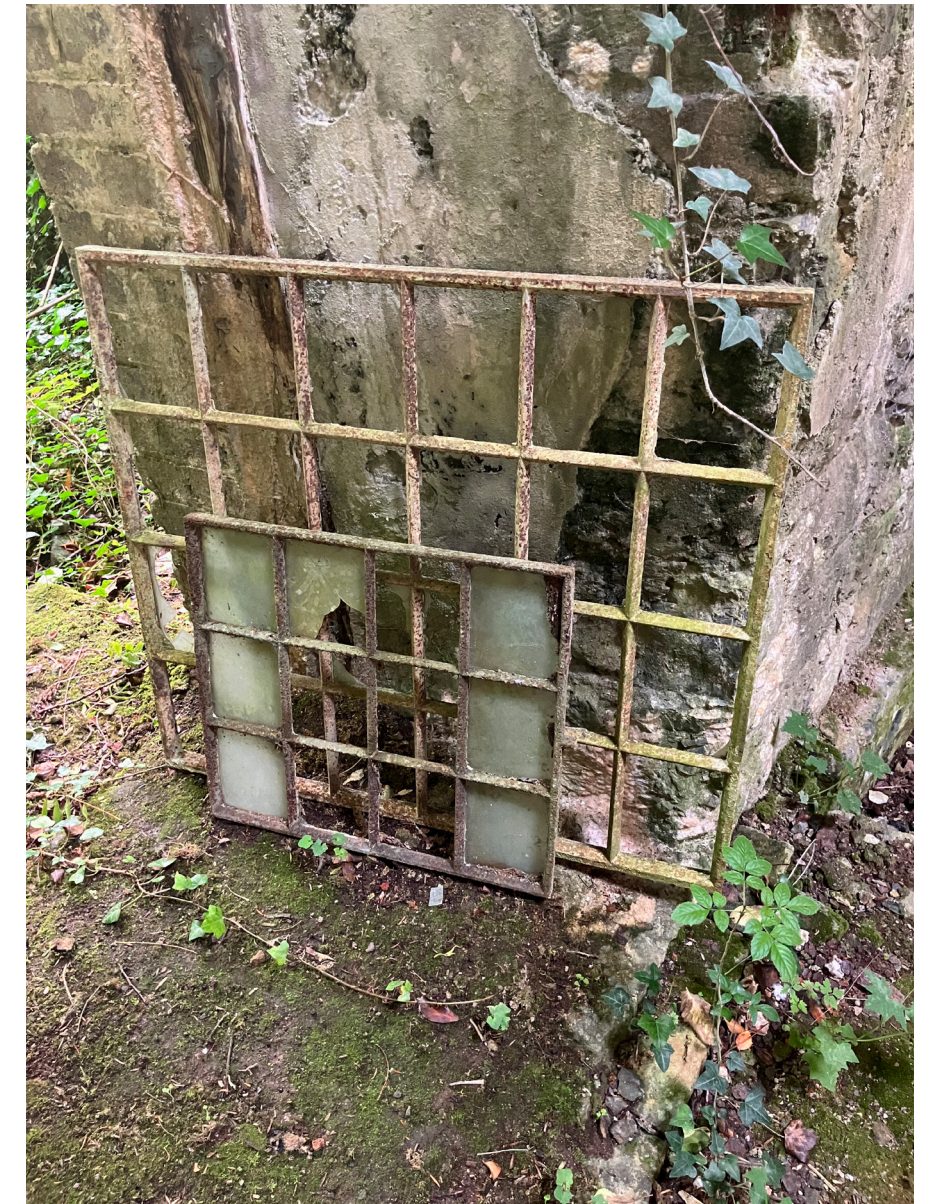
Figure 137 - Cast iron windows. in still house.
