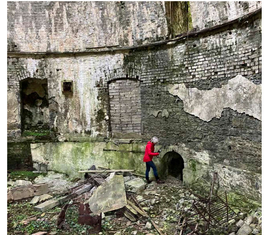
Figure 44 - Mash house general view of the interior looking north.
