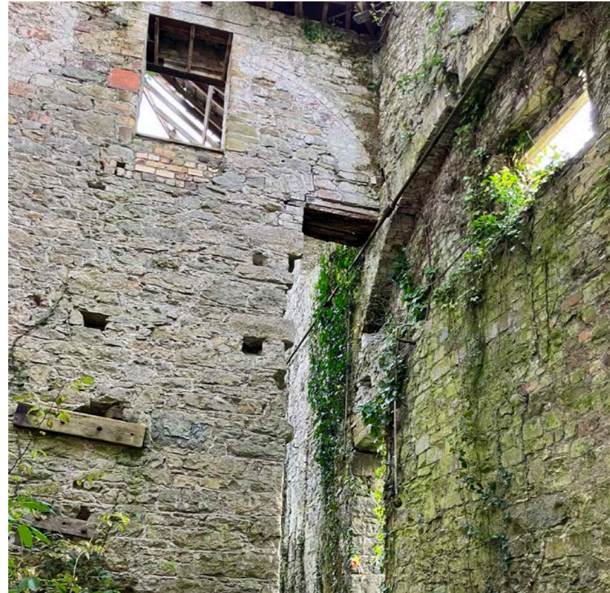
Figure 72 - Kiln/engine house interior view of chimney.
