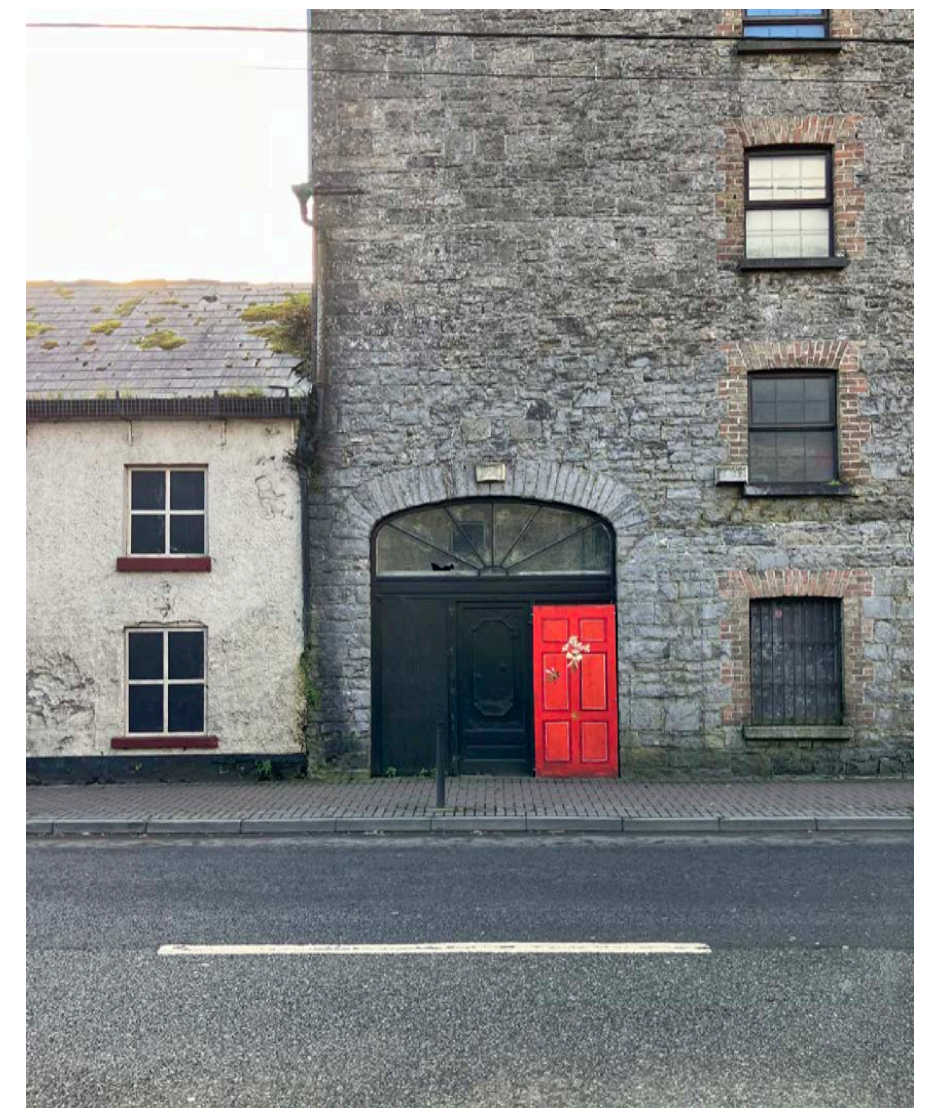
Figure 93 - Mill & grain store - infilled carriage arch.
