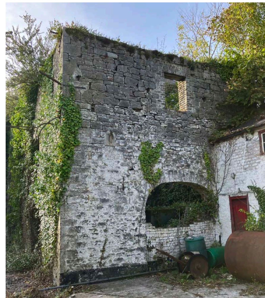
Figure 37 - Former engine house connection with near of offices building.
