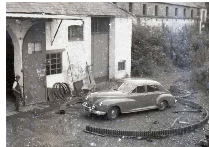
Figure 20 - Heavy shop looking towards the bonded warehouse in the 1960s.
