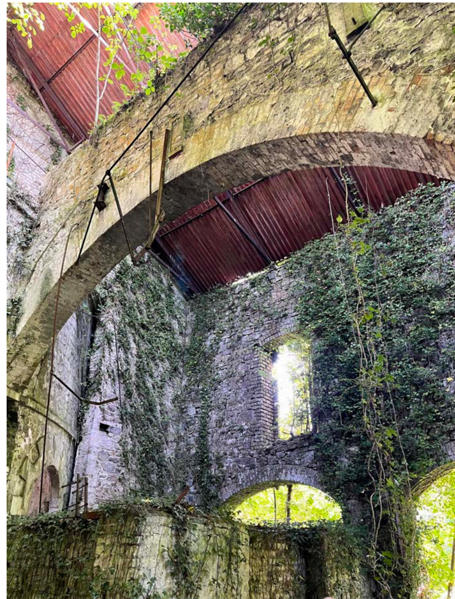
Figure 7 - Still house interior lookin East.
