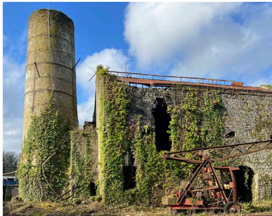
Figure 21 - Chimney on south side of still room.
