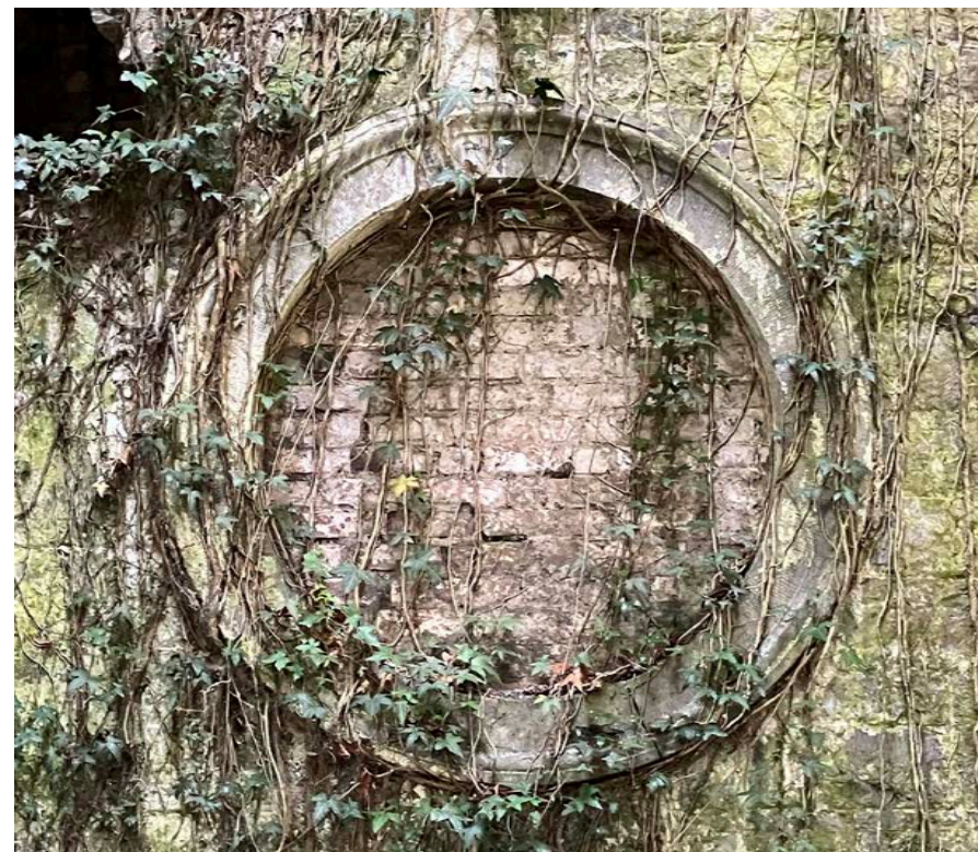
Figure 42 - Mash house detail of dressed stone decoration.
