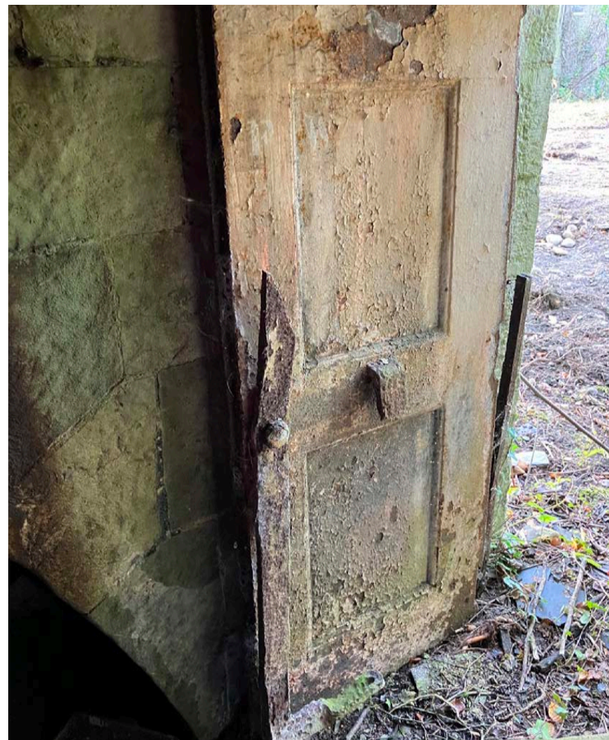
Figure 57 - Bonded warehouse detail of cast iron door
