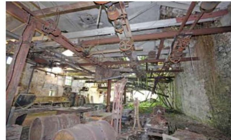
Fig.9 Overhead lineshafts in Building 2.
