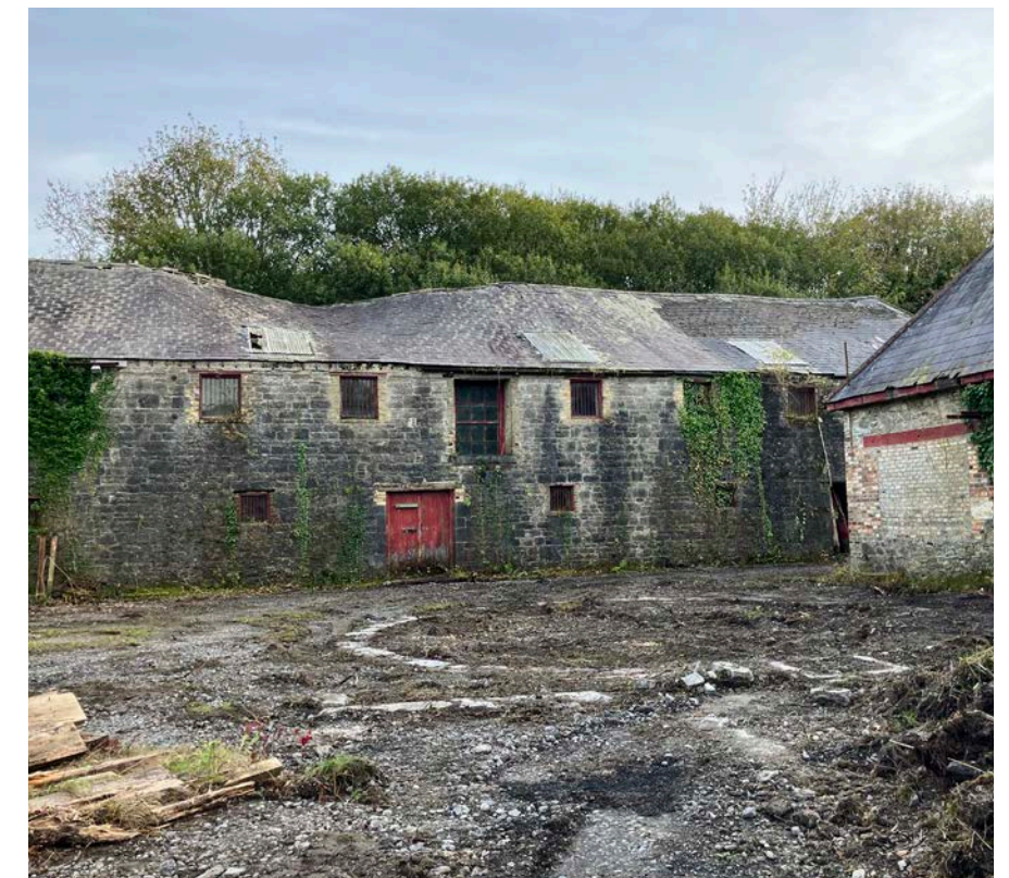
Figure 61 - Warehouse/cooperage from the west.
