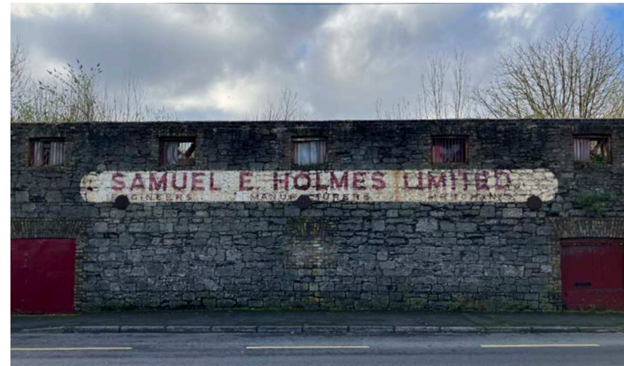
Figure 3 - Samuel E Holmes Ltd historic painted sign.
