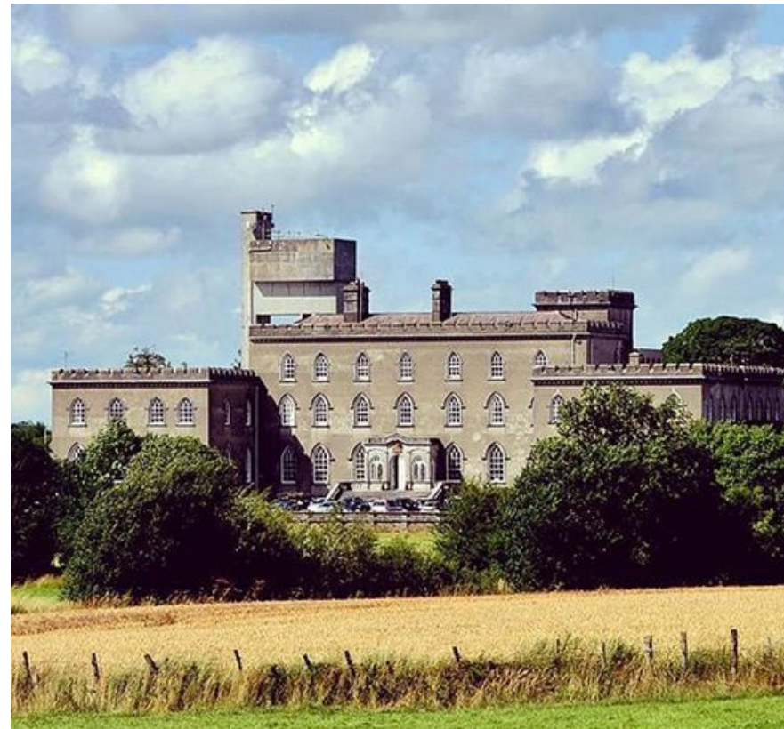
Figure 23 - View of Moore Abbey from the South.
