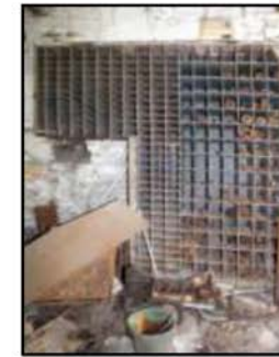
3. Pigeonhole racks along E side (1).
