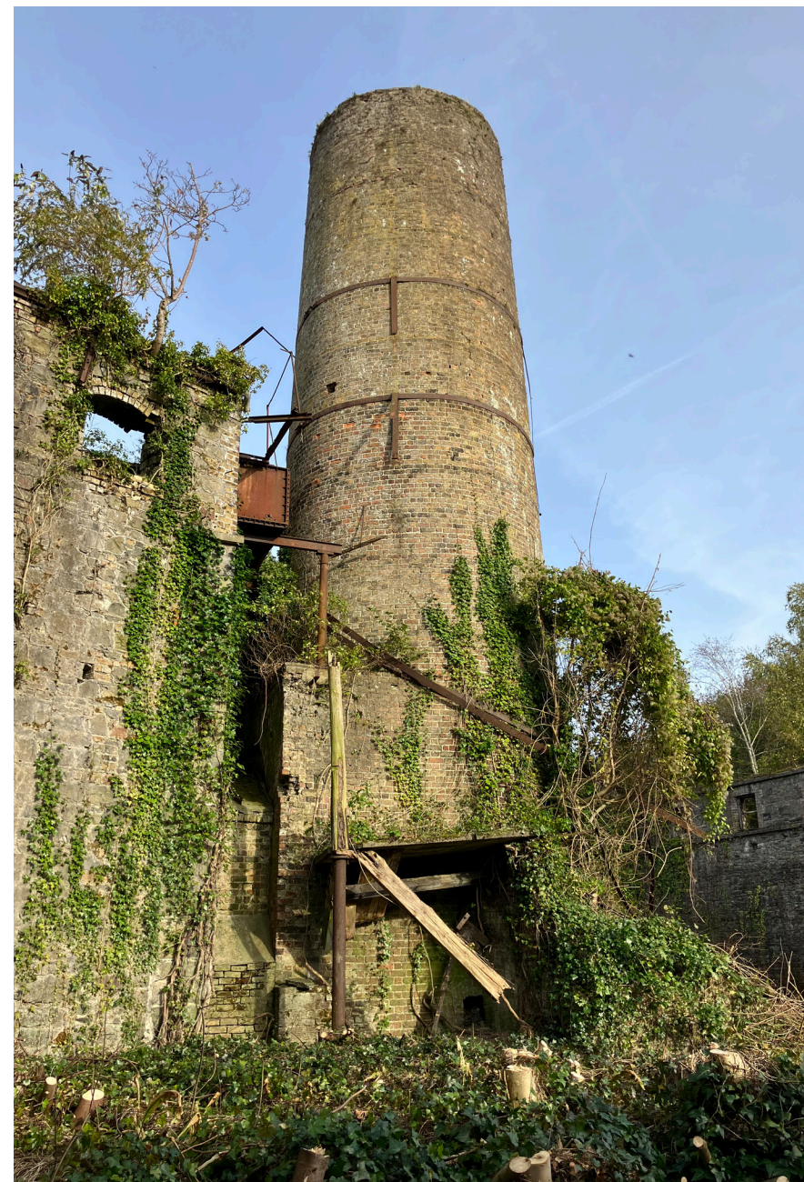
Figure 53 - Chimney on south side of still room.
