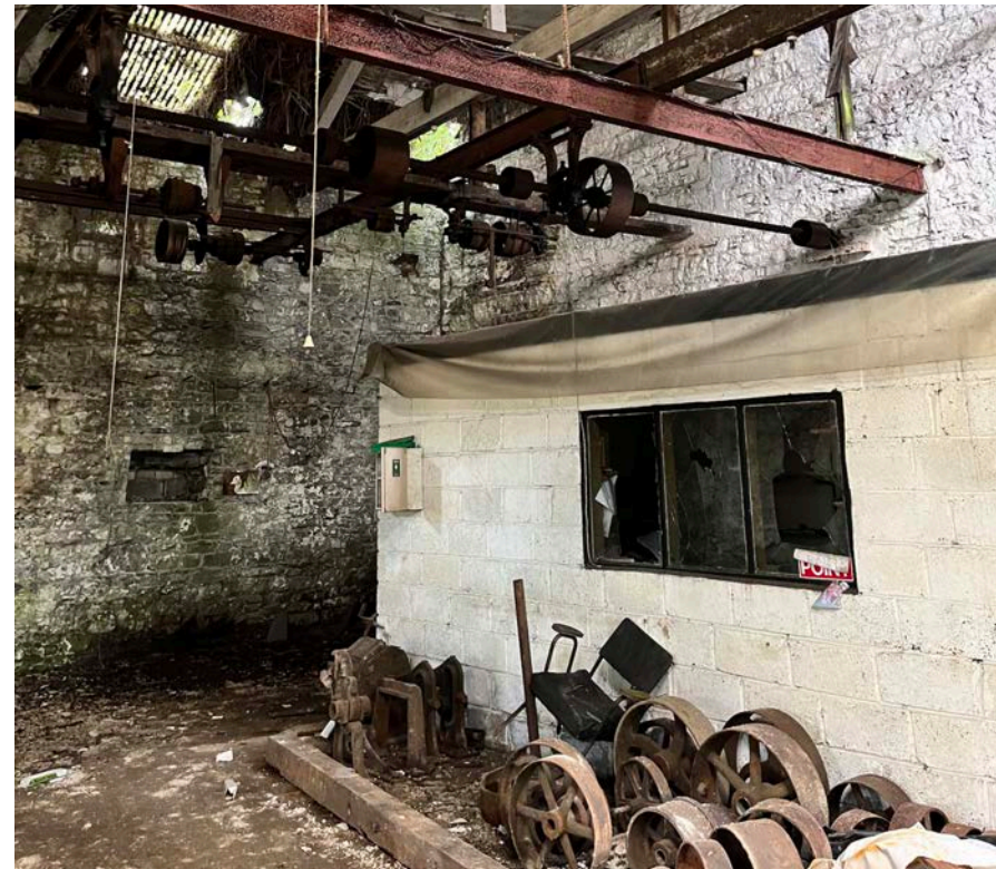
Figure 130 - Heavy shop office.
