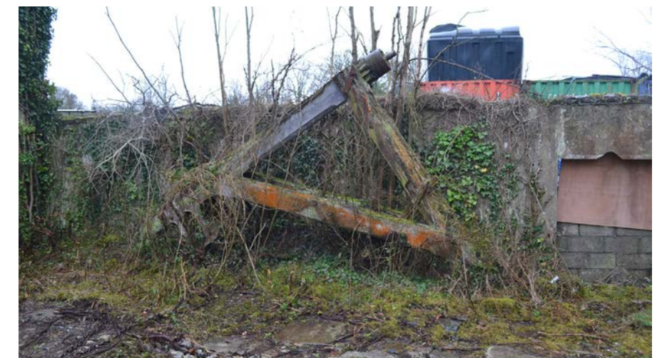
Figure 54 - Bonded warehouse - jib of former steam crane.
