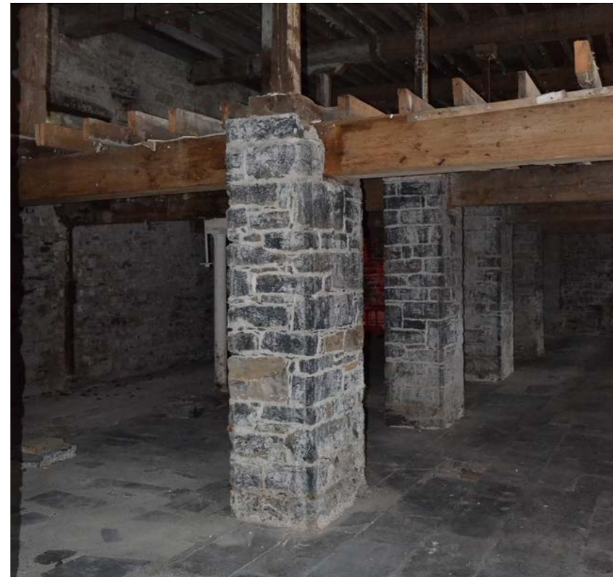
Figure 39 - Mill/grainstore ground floor structure & stone flagged floor.
