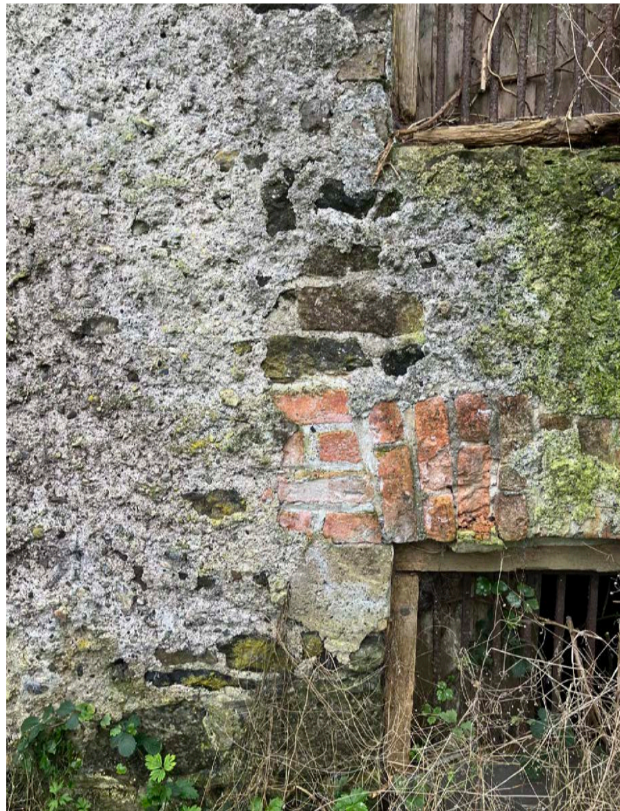
Figure 127 - Malt house detail of masonry and lime coating.
