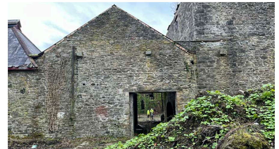
Figure 75 - The rubble stone east gable.
