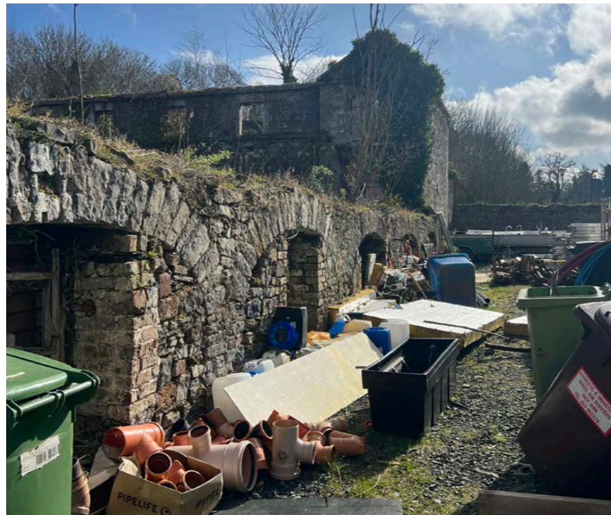
Figure 115 - Wall between former distillery and brewery yards
