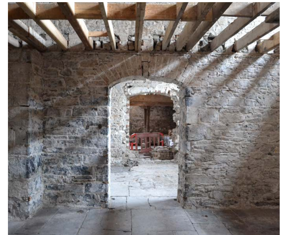
Figure 41 - Mill and grain store ground floor interior looking west.
