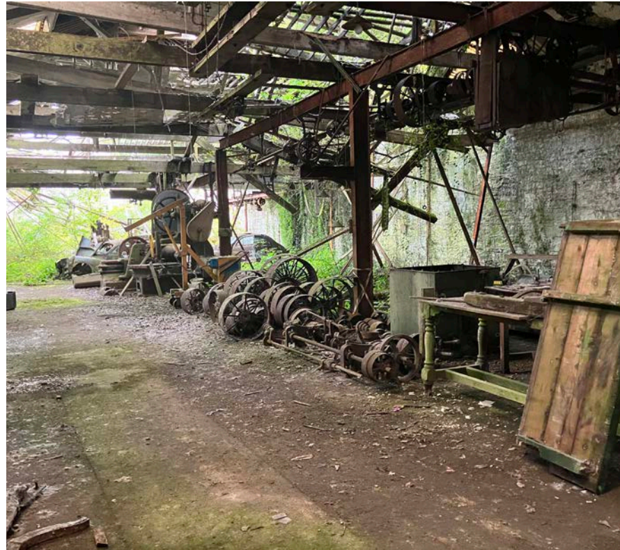
Figure 62 - Long shop interior looking East.
