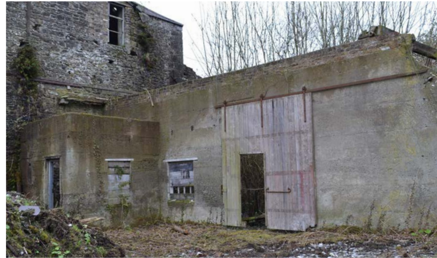
Figure 69 - Carpenter's shop remaining concrete walls.
