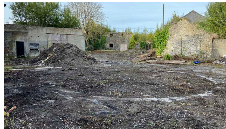
Figure 78 - Weighhouse external view. Gasometer base.
