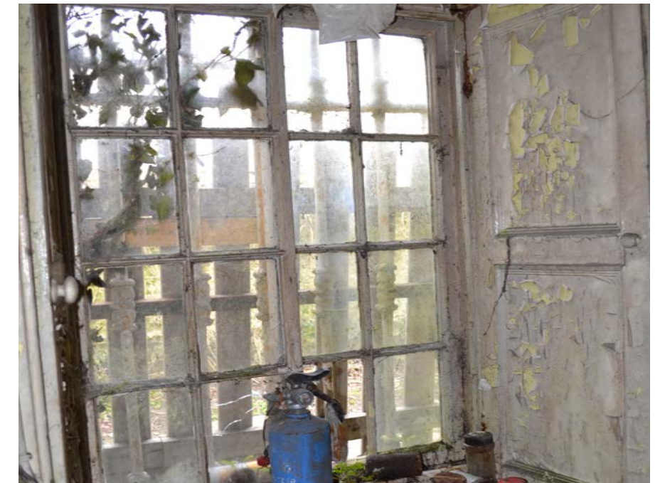
Figure 34 - Offices detail of original Yorkshire sash window
