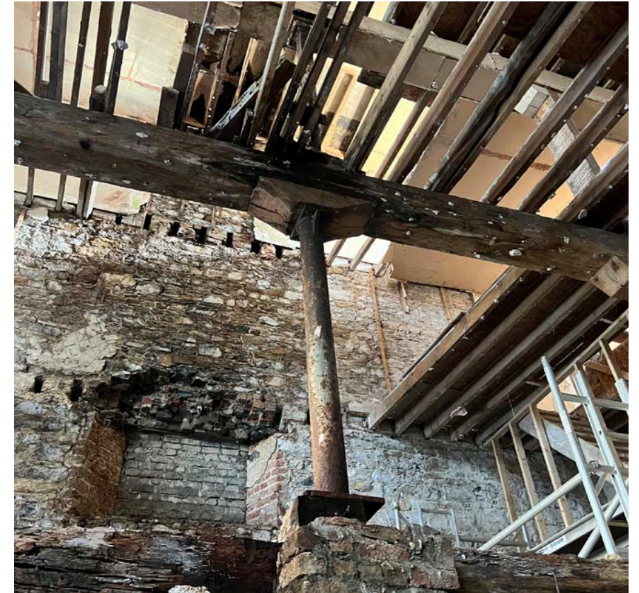
Figure 105 - Mill & grain store condition of internal floors.
