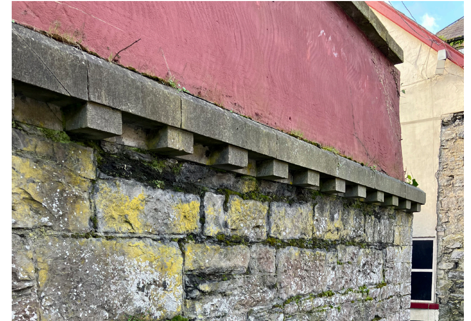
Figure 129 - Water tank - dressed stone dentil coping.
